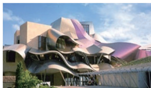
Fig. 1 View of a color-decorated building using an oxide-layered coating on titanium (Hotel Marquesde Riscal)
